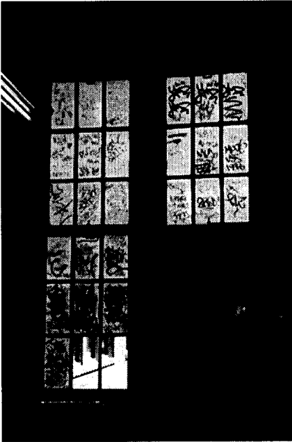
A school window is broken and covered by graffiti.
